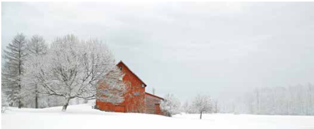
Above: Red Barn #5 , Charlotte, Vermont. Built early 1800s, this barn sits on the land that was once the Thomas Chittenden Orchard, the largest apple orchard in New England at the time. The structure was used as an apple processing barn.
